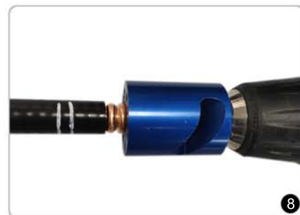
Using the low speed setting on the drill, insert exposed outer conductor into trimming tool base. Continue trimming until tool reaches cable jacket. Do not push tool beyond this point.
